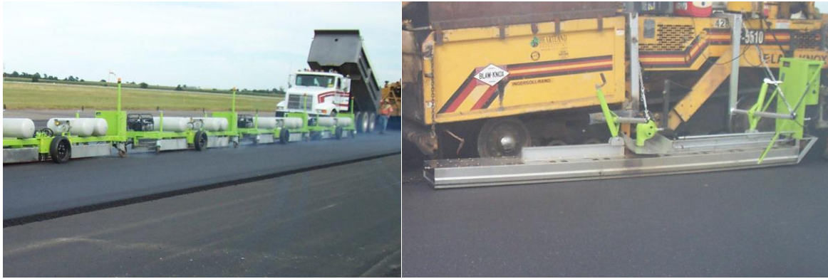
Figure 17. Large infra-red joint heater
