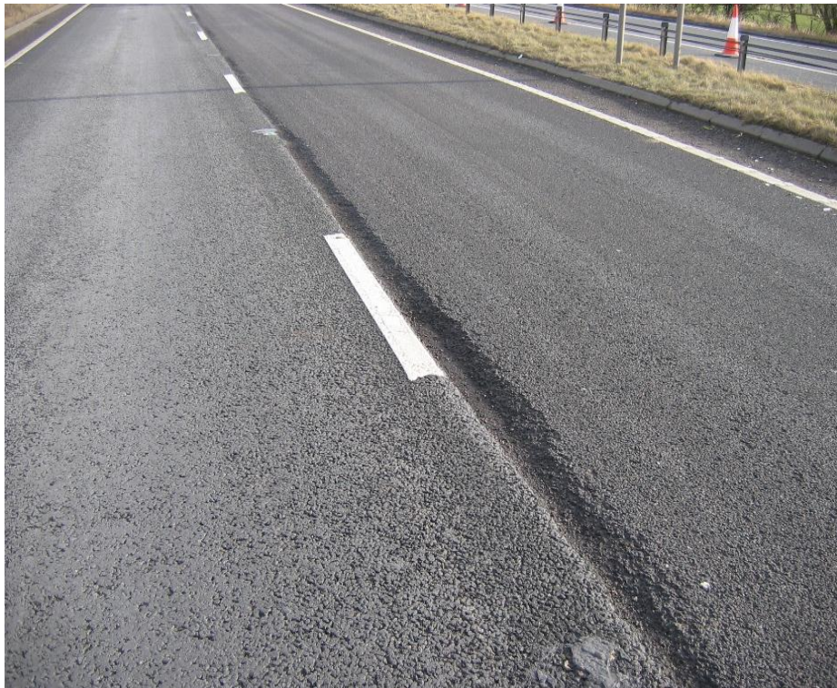
Figure 1 Fretting at a longitudinal joint in TSCS
