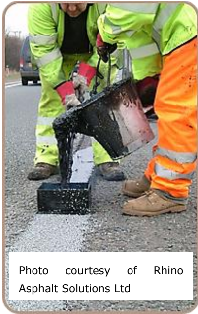
Figure 9. Pouring from bucket to shoe and using shoe
