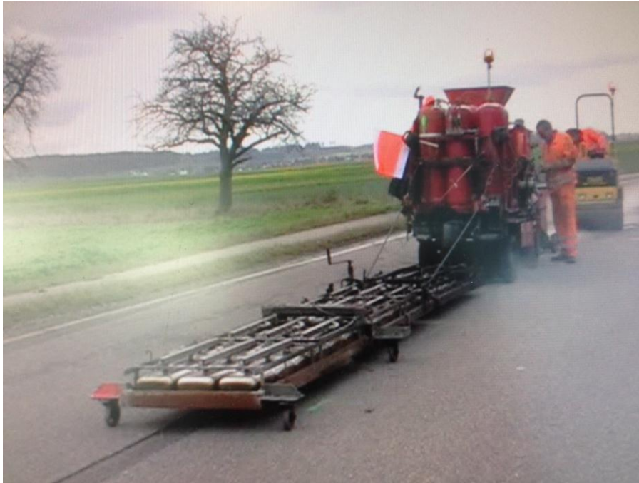
Figure 22. Infra-red heat and recycling system (photo courtesy of ASI)
