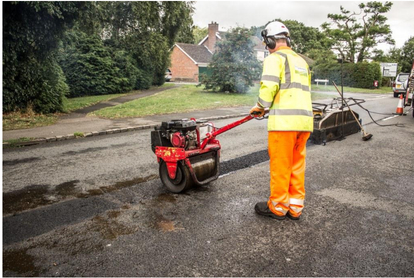
Figure 19. Joint repair procedure (photo courtesy of Nuphalt)
