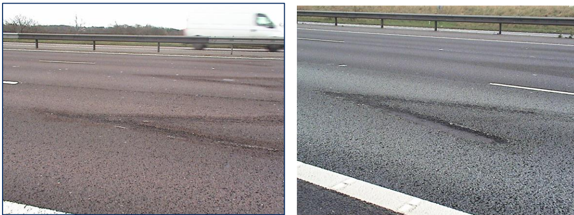
Figure 28 TSCS fretting as a result of 'burning off' road markings - HA Area 10
