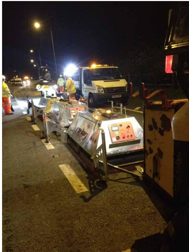
Figure 20. Infra-red heater units set up for joint repair (photo courtesy of Re-Lay Asphalt Services)
