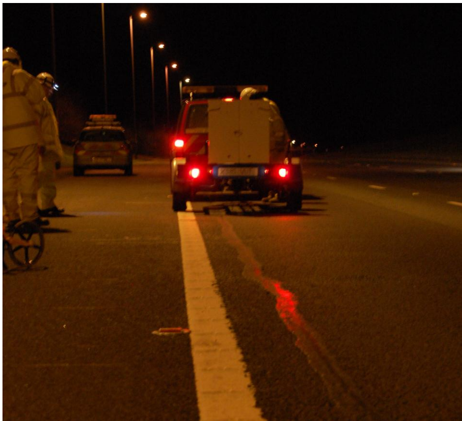
Figure 2 Sealed reflection type crack above a longitudinal joint in binder course
