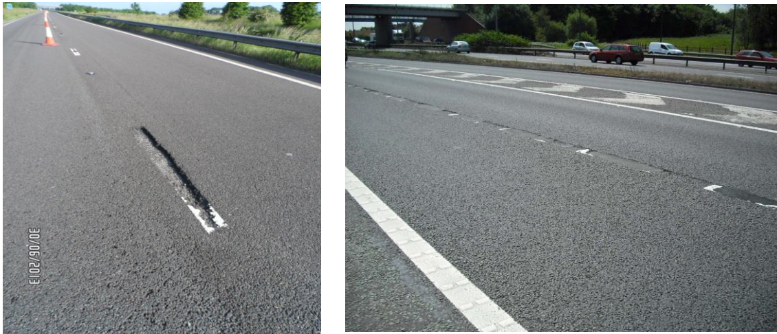
Figure 27 TSCS 'white line' failures – HA Areas 12 and 10 respectively
